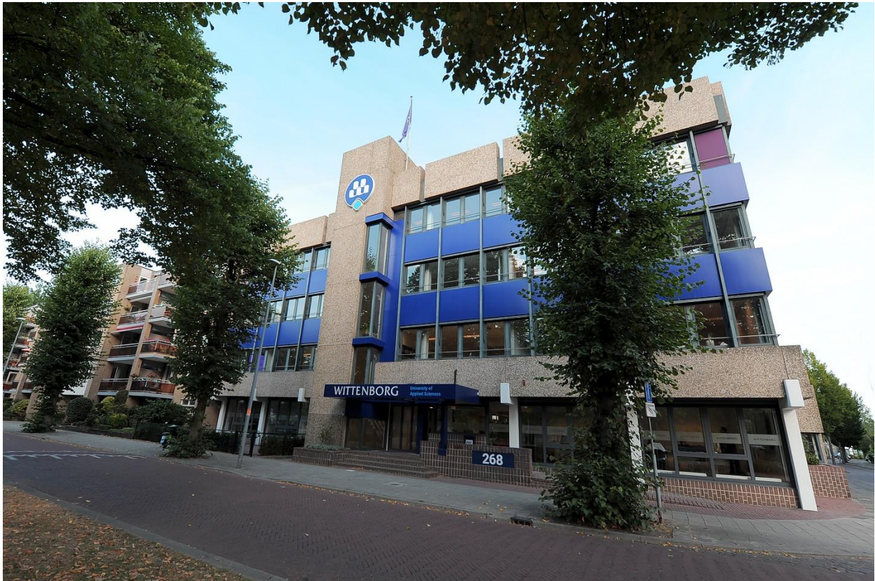
Wittenborg's Brinklaan Building, Apeldoorn
